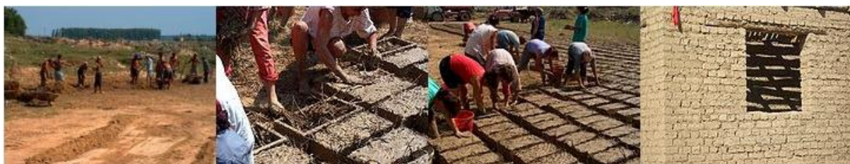
Adobe soil collection Moulding into bricks Sun-drying of bricks Adobe house
