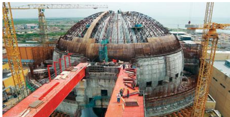
Figure 9 Nuclear power dome construction at Kaiga, India
