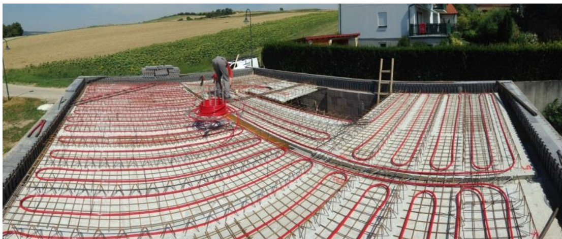
Figure 3 Demonstration house in Austria using the ceiling for energy storage [9]
