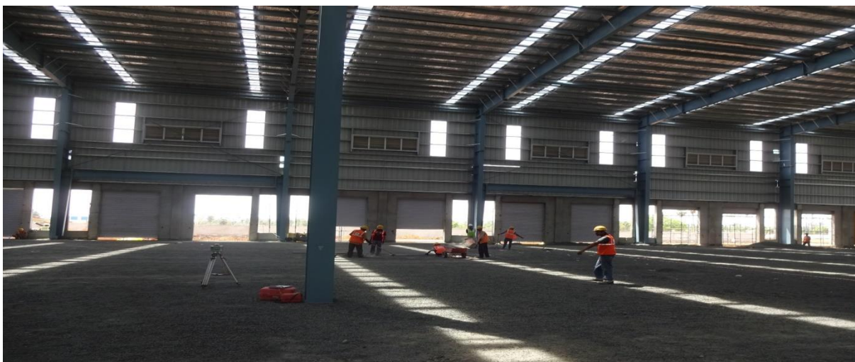
Figure 1 Shows the sub base preparation in progress.
