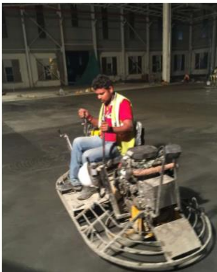
Figure 6 The Power floater in Progress to remove imperfection in floor
