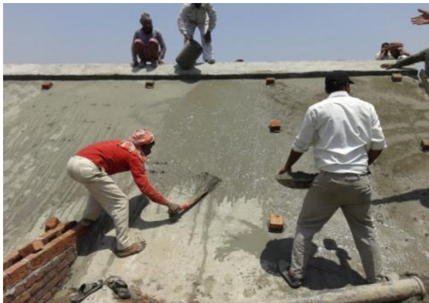
Fig. 6 Placement of lightweight concrete for roof insulation
