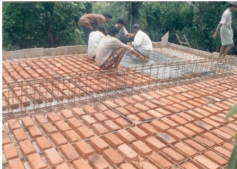
Figure 1 A RC filler-slab roof being constructed with bricks as fillers
