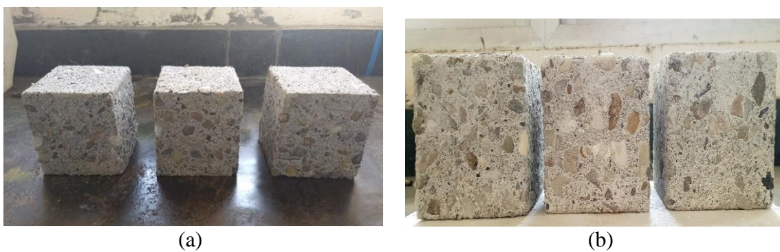
Figure 5 Deteriorated surface of (a) NS based concrete and (b) MS based concrete after immersion in H 2 SO 4 solution
